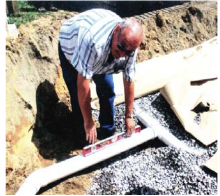
Doug Metson, Chief Building Inspector, verifies the proper specifications for this new septic system.
